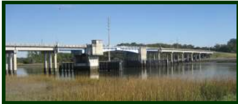
Original Draw Bridge Serving Skidaway: 1972-2014
